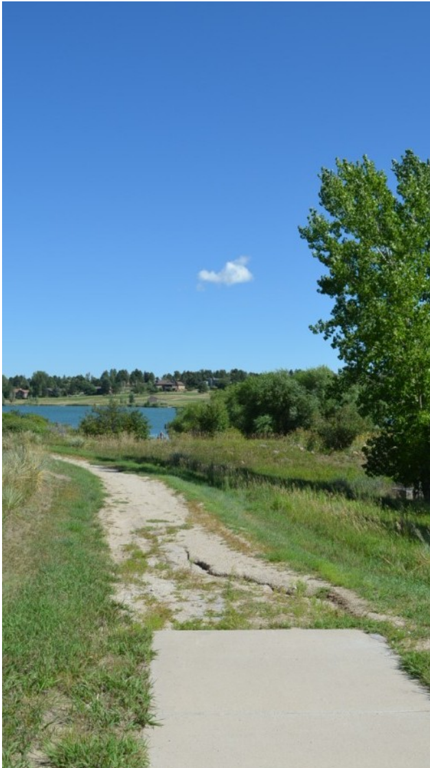
View Northward at South starting point of the new concrete trail project, at the end of the existing concrete.
