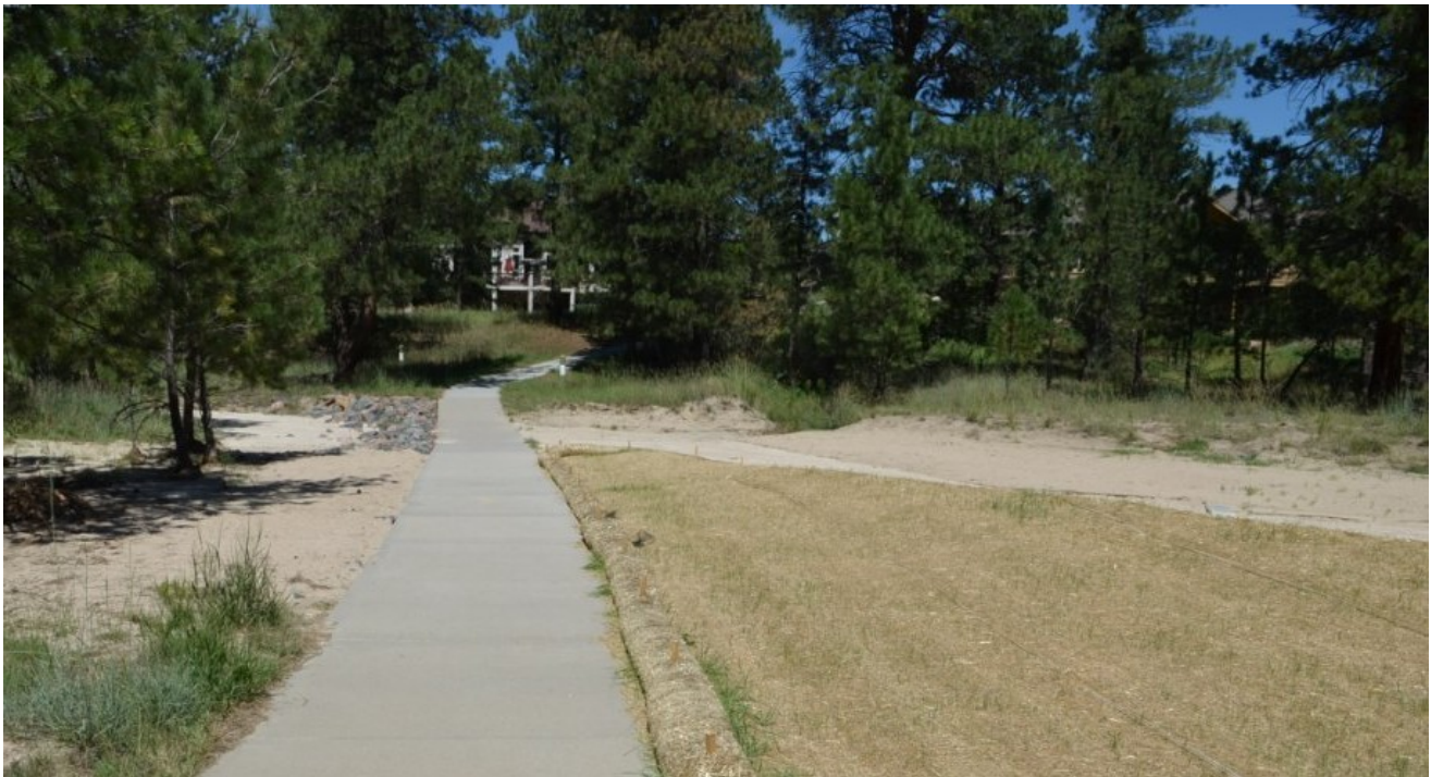
Texas-Crossing Improvements and Erosion protection
