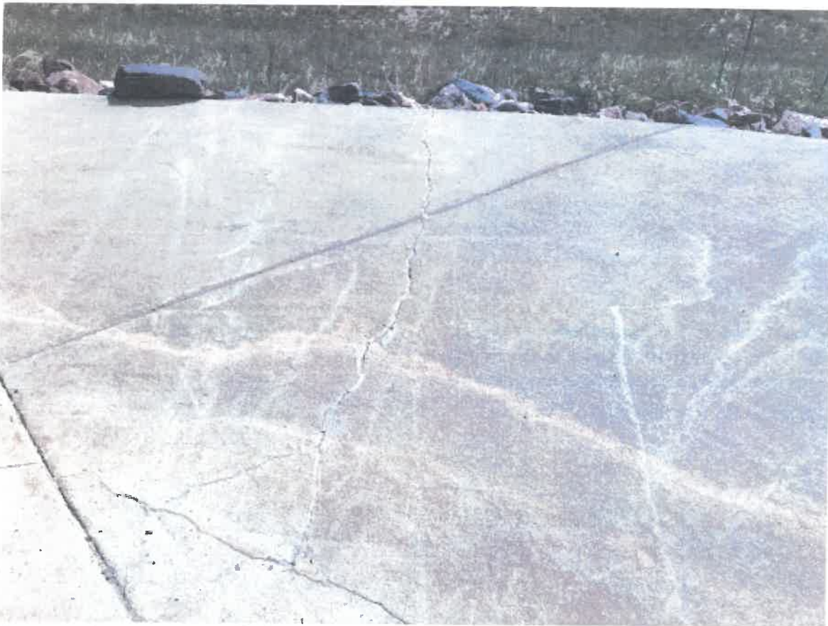
Photograph 4: Repair cracks in concrete at forebay.
